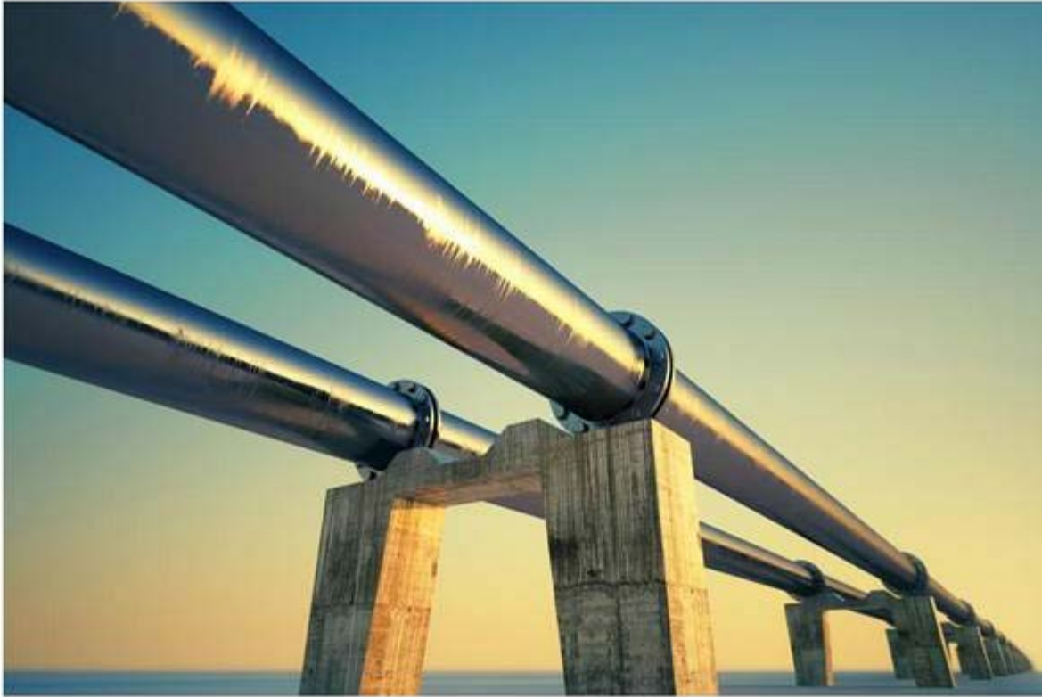
Serious pipeline incidents dropped 70 percent over the last 10 years, according to data from the Pennsylvania Public Utility Commission.
